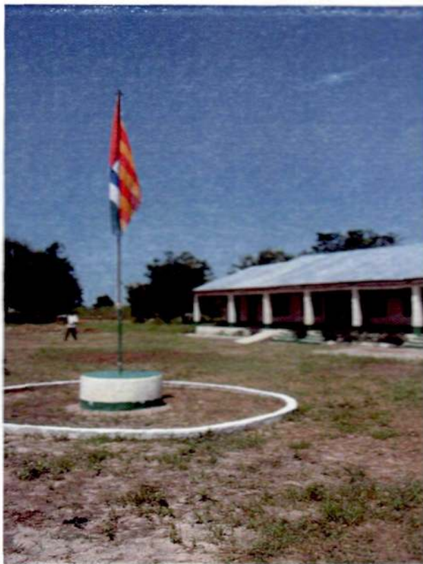
BAJA KUNDA SCHOOL BUILDING BLOCK A
