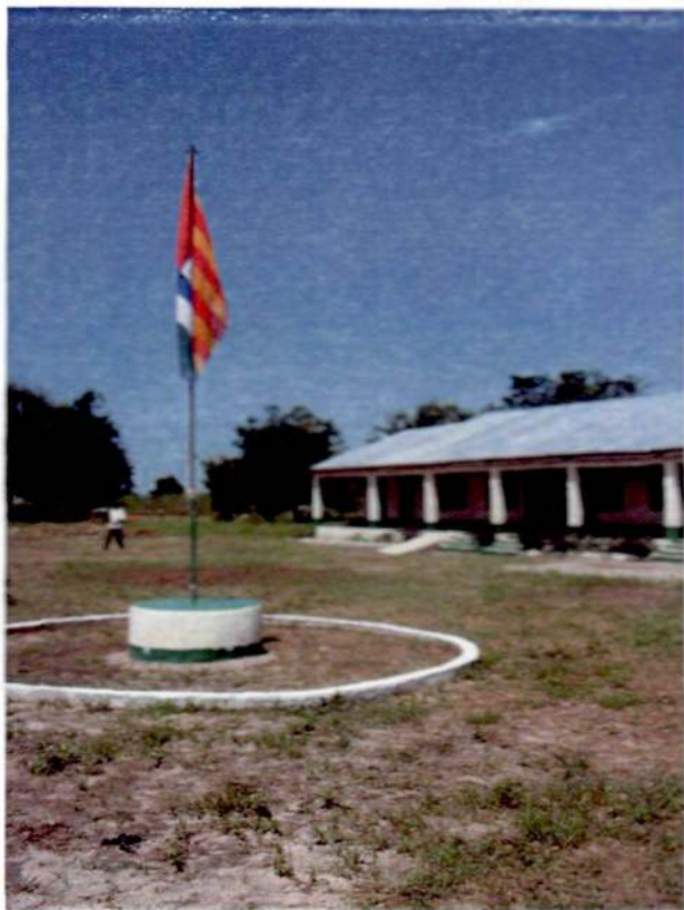
BAJA KUNDA SCHOOL BUILDING BLOCK A
